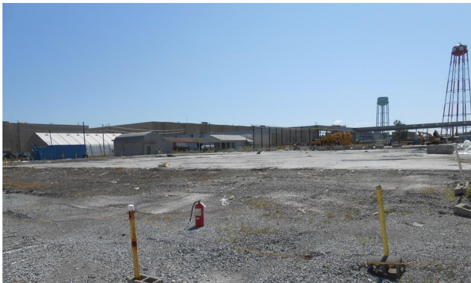
Figure 14. C-410/420 slab after demolition
