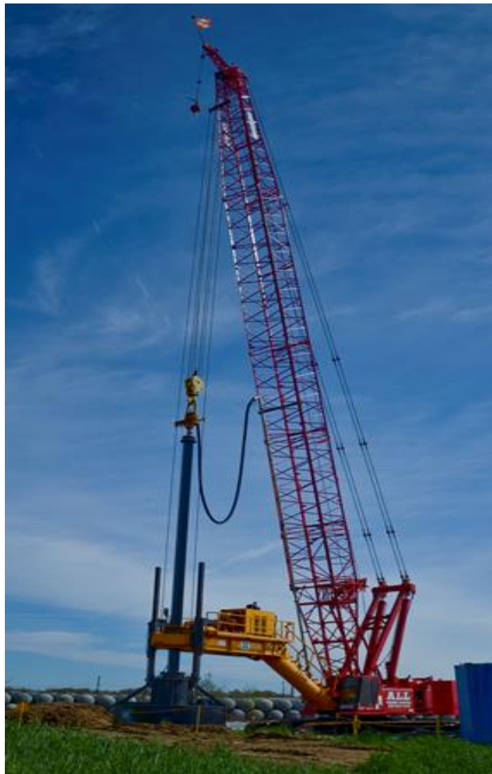
Figure 12. Deep Soil Mixing at SWMU 1
